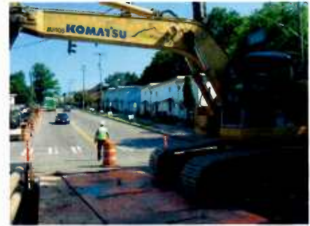
Construction of the First Hill Streetcar. Photo provided by Nebiyou Abunie.
