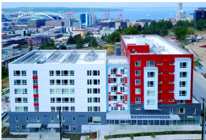
The rooftop of Hoa Mai Gardens, showing solar panels used to pre-heat water for the building.
