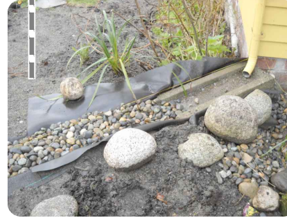
DOWNPOUT TO RAIN GARDEN ROCK TRENCH CONNECTION
