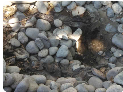
DISPERSION TRENCH WITH OVERFLOW ARMORING
