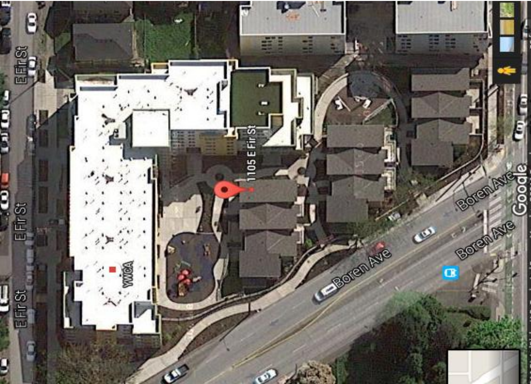
Area of responsibility includes ROW along Boren, Yesler and Fir Street; interior courtyards.
