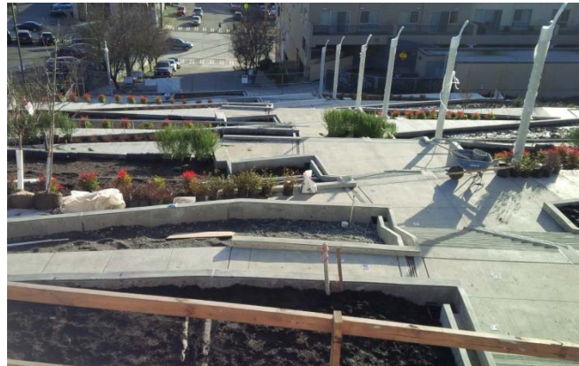
In 2015, the concrete stairs and ramps were poured for the 10 th Ave S Hillclimb.
