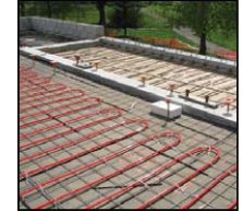
Hydronic heating/cooling w/ district energy.
