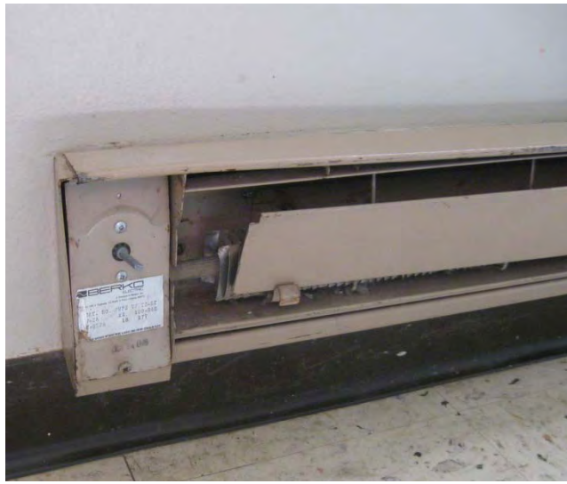
Photo 6 Electric Baseboard Heater with Panel Cover
