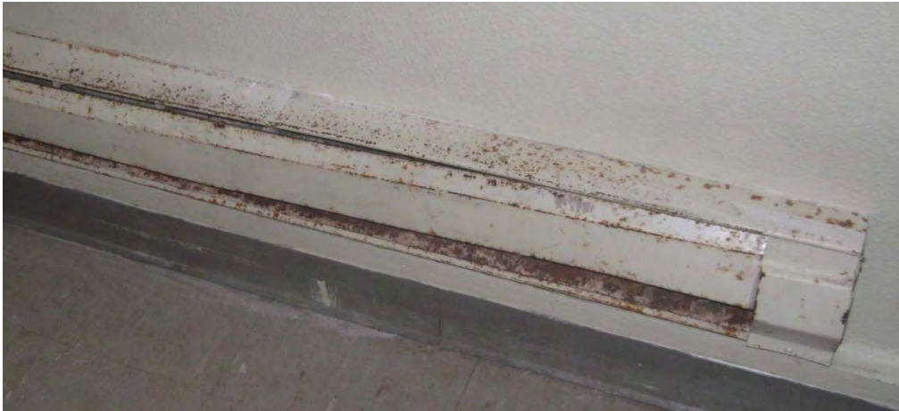
Photo 4 Baseboard Heater in Poor Condition
