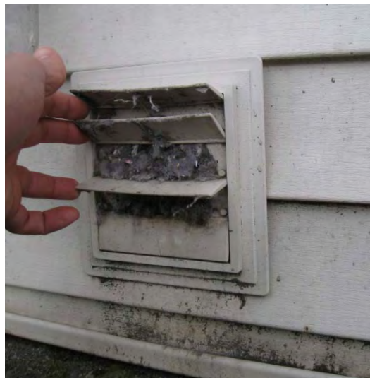
Photo 3 Dryer Exhaust Termination with Lint Build-up
