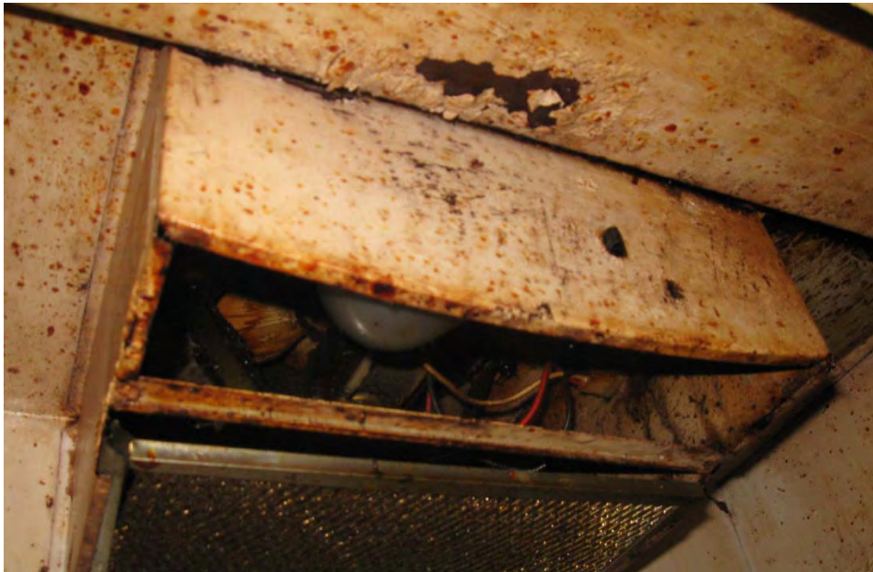
Photo 5 Kitchen Rangehood Exhaust Fan
