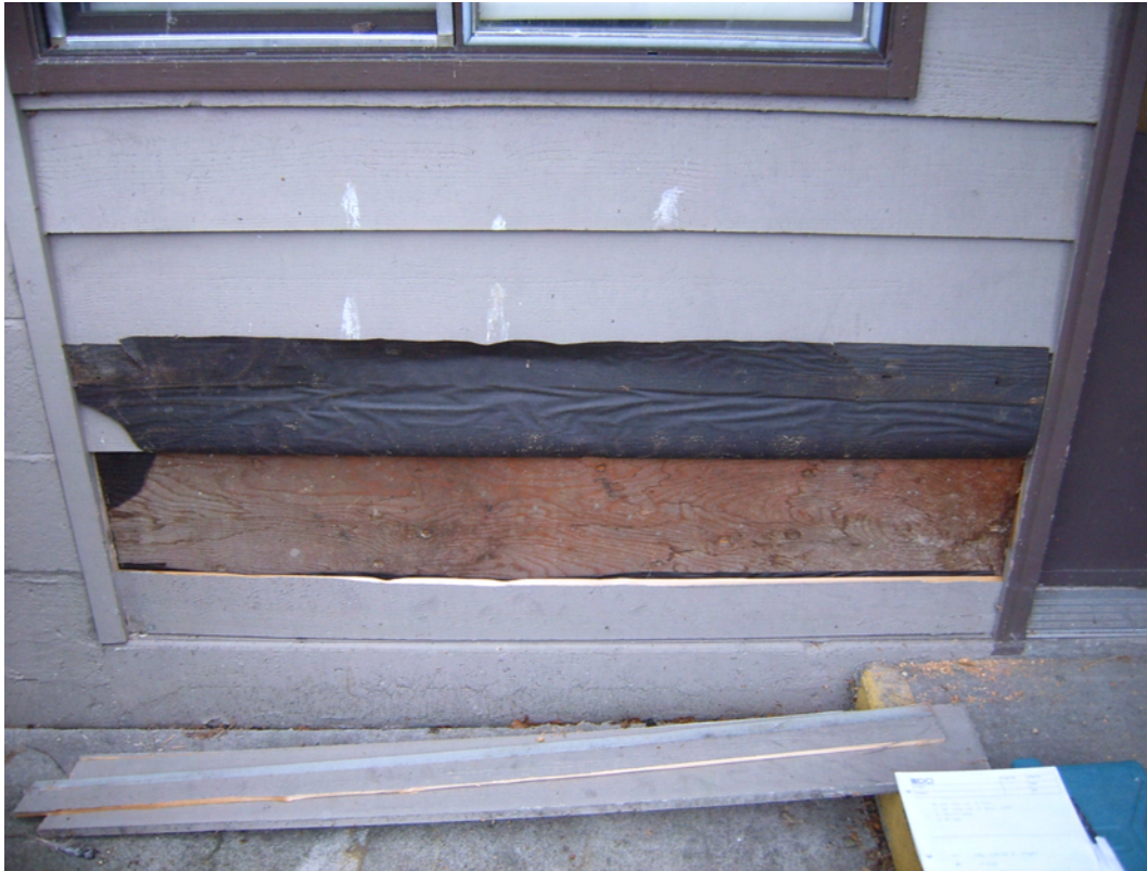
Photograph #5 – Inadequate Exterior Sheathing Attachment
