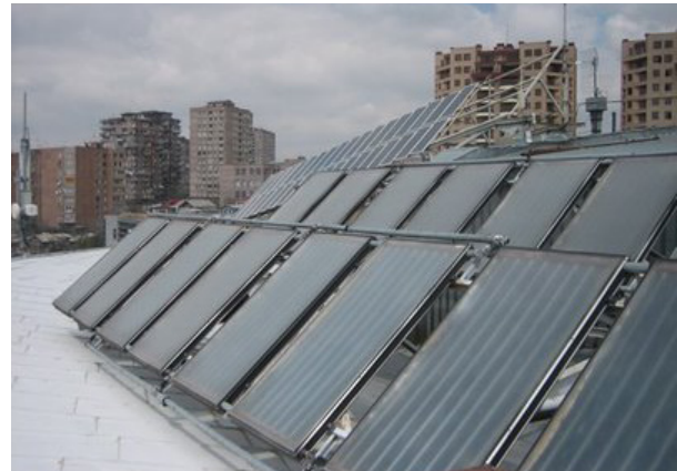
Figure 5: Photo of an Installed Bank of Roof-Mounted Solar Panels
