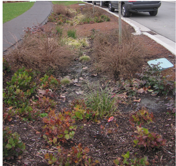
Figure 10: A Vegetative Swale Design
