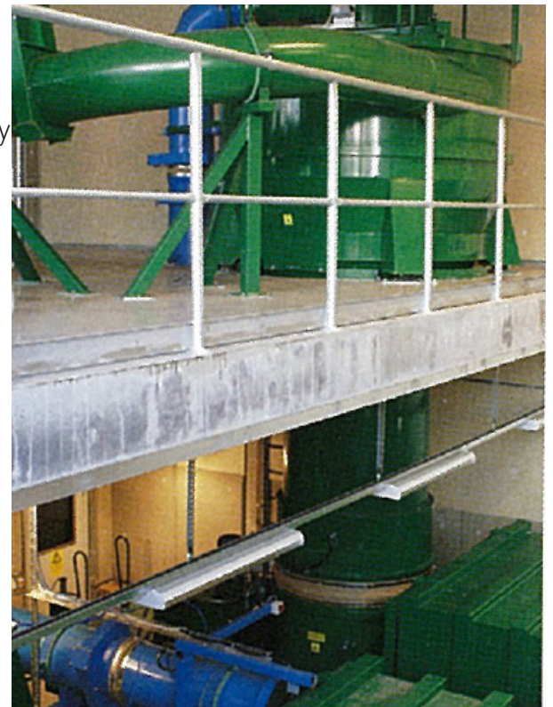
Pneumatic waste disposal system. All refuse chutes are linked by underground pipes to a central collection station. An advanced control system at the station sorts waste into the appropriate container. (Novotny)
