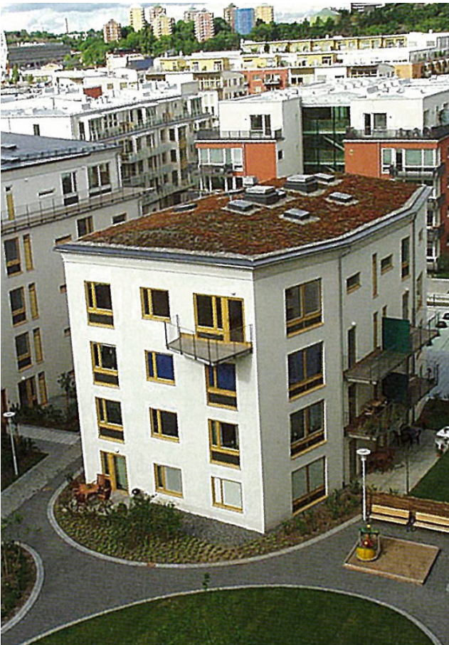
Green roofs on some buildings in Sjöstaden are another link in the local stormwater treatment chain. (Novotny)
