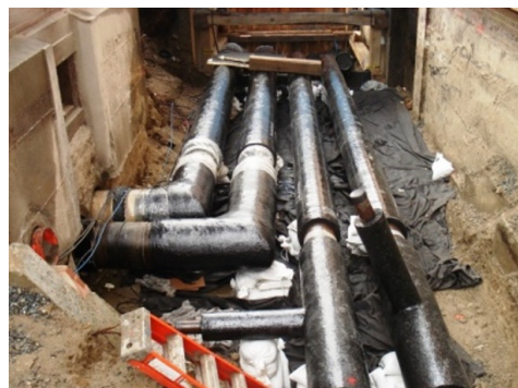
Figure 7: Photo of A Partially-Installed Four-Pipe CCHP Distribution System
