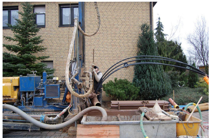
Typical equipment for drilling a vertical-bore well. From www.erdwaerme-zeitung.de/images/sondeneinbau
