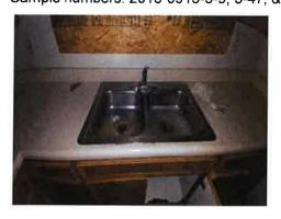
There is a total of six (6) aluminum sinks with asbestos containing black undercoating located in rooms 3, 12, 20, 36, 44, & 52 of building #20.
