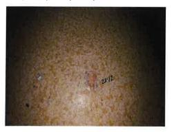
There is approximately 325 square feet of asbestos-containing white backing with mastic associated with tan sheet vinyl flooring located in rooms 7, 13, 19, 31, 42, 49, 54, 74, 79 of building #21. The substrate is wood.
