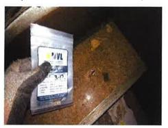
There is approximately 60 square feet of asbestos-containing white backing with mastic associated with brown sheet vinyl flooring / steps located in room 7, 14 of building #22. The substrate is wood.
