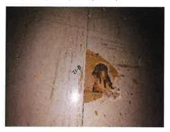
There is approximately 2340 square feet of asbestos-containing white / beige vinyl floor tiles located under vinyl floor tiles in rooms 3, 9, 10, 11, 14, 15, 17, 18, 20, 21, 23, 24, 25, 34, 36, 51, 52, 53, 55, 56, 58 of building #21. The associated mastic is not asbestos containing. The substrate is wood.
