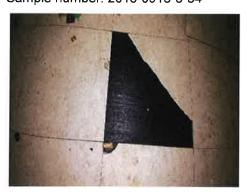
There is approximately 235 square feet of asbestos-containing black floor mastic associated with white vinyl tiles in rooms 33 & 35 of building #21. The substrate is wood.
