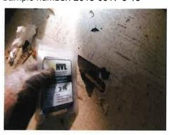
There is approximately 70 square feet of asbestos-containing black floor mastic associated with white vinyl floor tiles in rooms 14 of building #22. The substrate is wood.
