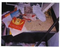
There is approximately 95 square feet of asbestos-containing off-white backing with mastic associated with tan sheet vinyl flooring located on the shelf in room 5 & 13 and in room 8 (under beige sheet vinyl) of building #19. The substrate is wood.
