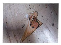
There is approximately 370 square feet of asbestos-containing white / beige vinyl floor tiles with black mastic located under vinyl floor tiles in rooms 1, 12, 32, 34, & 43 of building #21. The substrate is wood.
