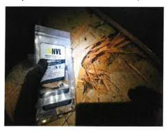
There is approximately 635 square feet of asbestos-containing beige vinyl floor tiles located under white vinyl floor tiles in room 1, 5, 6, 20, 23, 24 of building #22. The associated mastic is not asbestos containing. The substrate is wood.
