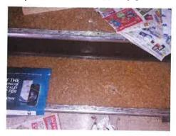
There is approximately 75 square feet of asbestos-containing off-white backing with tan mastic associated with brown sheet vinyl flooring / steps located in room 1 & 9 of building #19. The substrate is wood.
