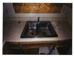
There is a total of twelve (12) aluminum sinks with asbestos containing black undercoating located in rooms 3, 8, 14, 20, 27, 32, 43, 50, 55, 61, 67, 75 of building #21.
