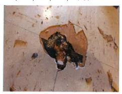
There is approximately 1,580 square feet of asbestos-containing brown / tan / beige vinyl floor tiles located under vinyl floor tiles in rooms 2, 9, 11, 13, 14, 15, 17, 19, 21, 22, 23, & 59 of building #20. The associated black mastic is not asbestos containing. The substrate is wood.
