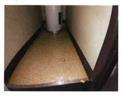
There is approximately 365 square feet of asbestos-containing off-white backing with mastic associated with beige sheet vinyl flooring located on the shelf in rooms 4, 13, 21, 53, 61 and on the floor in rooms 8, 24, 40, 48, 56, & 64 of building #20. The substrate is wood.
