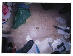
There is approximately 300 square feet of asbestos-containing beige vinyl floor tiles located in room 5 thru 7 of building #19. The associated black mastic is not asbestos containing. The substrate is wood.
