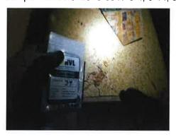
There is approximately 105 square feet of asbestos-containing white backing with mastic associated with tan sheet vinyl flooring located in room 3, 9, 21 of building #22. The substrate is wood.
