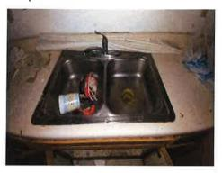
There is a total of three (3) aluminum sinks with asbestos containing black undercoating located in room 5, 14, and 30 of building #18.
