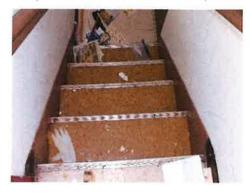
There is approximately 140 square feet of asbestos-containing white backing with black mastic associated with brown sheet vinyl flooring / steps located in room 3, 11, 19, and 27 of building #18. The substrate is wood.
