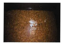
There is approximately 140 square feet of asbestos-containing off-white backing with mastic associated with brown sheet vinyl flooring / steps located in rooms 1, 25, 48 & 78 of building #21. The substrate is wood.
