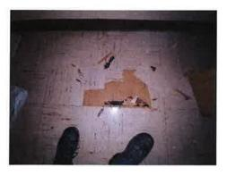
There is approximately 570 square feet of asbestos-containing beige / brown / tan vinyl floor tiles with black mastic located under vinyl floor tiles in room 33, 49, 51, 53, 54, & 55 of building #20. The substrate is wood.
