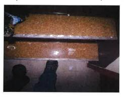
There is approximately 255 square feet of asbestos-containing off-white backing with mastic associated with brown sheet vinyl flooring / steps located in rooms 1, 9, 17, 33, 41, 49 & 57 of building #20. The substrate is wood.
