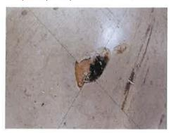
There is approximately 900 square feet of asbestos-containing beige vinyl floor tiles located under 12x12 white vinyl tile flooring in room 3, 11, 12, 13, 15, 16, 17, 19, and 23 thru 25 of building #18. The associated mastic is not asbestos containing. The substrate is wood.
