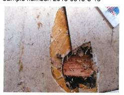
There is approximately 175 square feet of asbestos-containing 12x12 white vinyl floor tiles located in room 7, 8, and 9 of building #18. The associated mastic is not asbestos containing. The substrate is wood.
