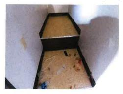
There is approximately 200 square feet of asbestos-containing backing with mastic associated with cream sheet vinyl flooring and shelf flooring located in room 6 (closet), 15, 23, 31, 32, and under tan sheet vinyl in room 10 & 18 of building #18. The substrate is wood.
