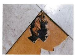
There is approximately 140 square feet of asbestos-containing beige vinyl floor tiles with black mastic located under 12x12 white vinyl tile flooring in room 6 (including the closet) of building #18. The substrate is wood.
