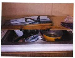
There is a total of four (4) aluminum sinks with asbestos containing black undercoating located in room 4, 12, 20, and 27 of building #19.
