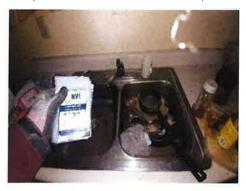
There is a total of six (6) aluminum sinks with asbestos containing black undercoating located in room 4, 10, 17, 22, 28, 34 of building #22.
